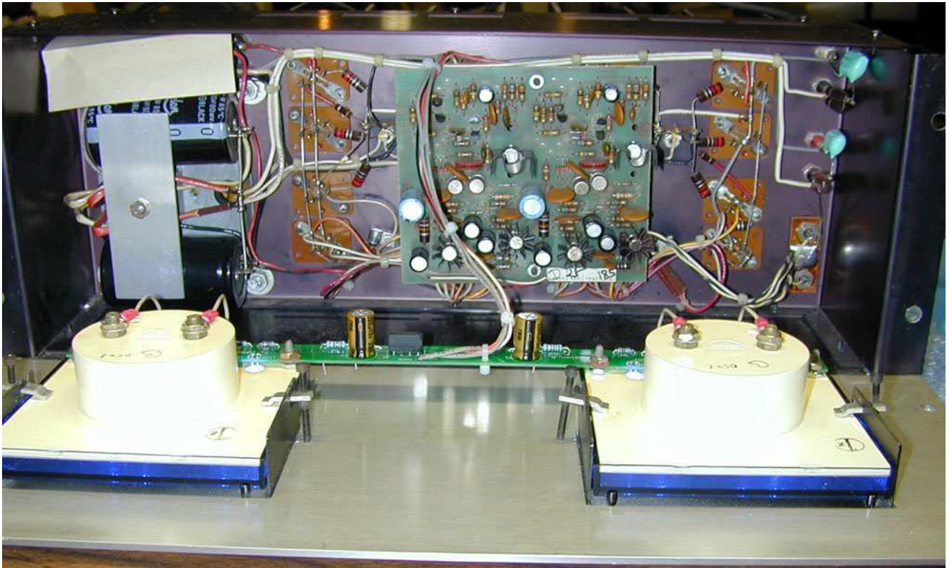
Figure 11 Installed LED Light Board Assembly
